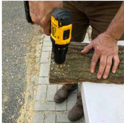
LEFT: Drill two holes instead of one, when using a wide base, lends more stability to the swing.
