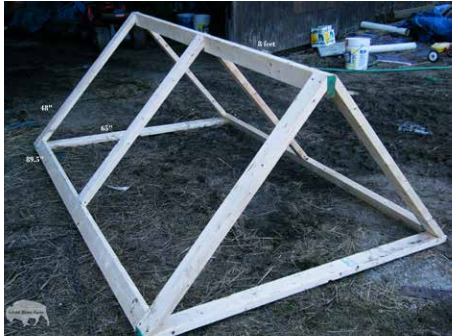
The frame is made out of eight 2x4s.
